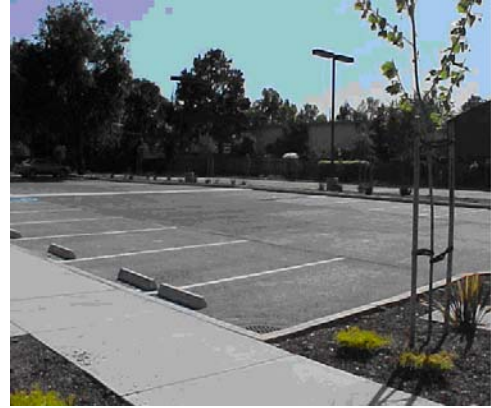
Porous-paved parking lot: a stormwater site design and treatment control measure.
