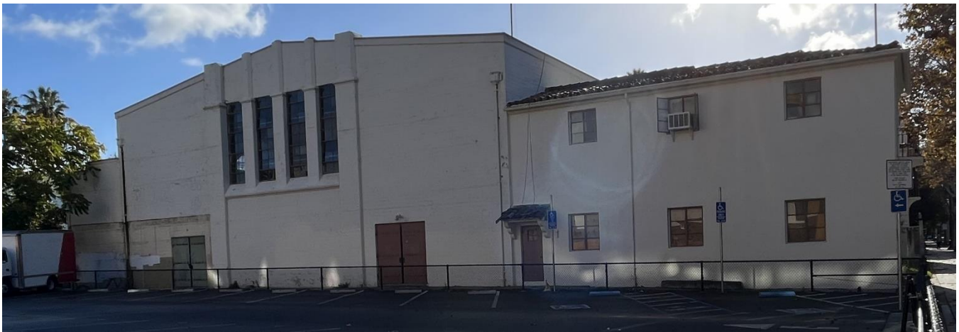
Figure 5. The north façade of 240 N. Second Street.
