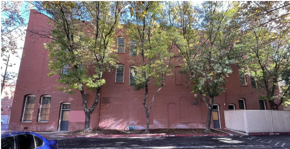
Figure 8. The west façade of 227 N. First Street.
