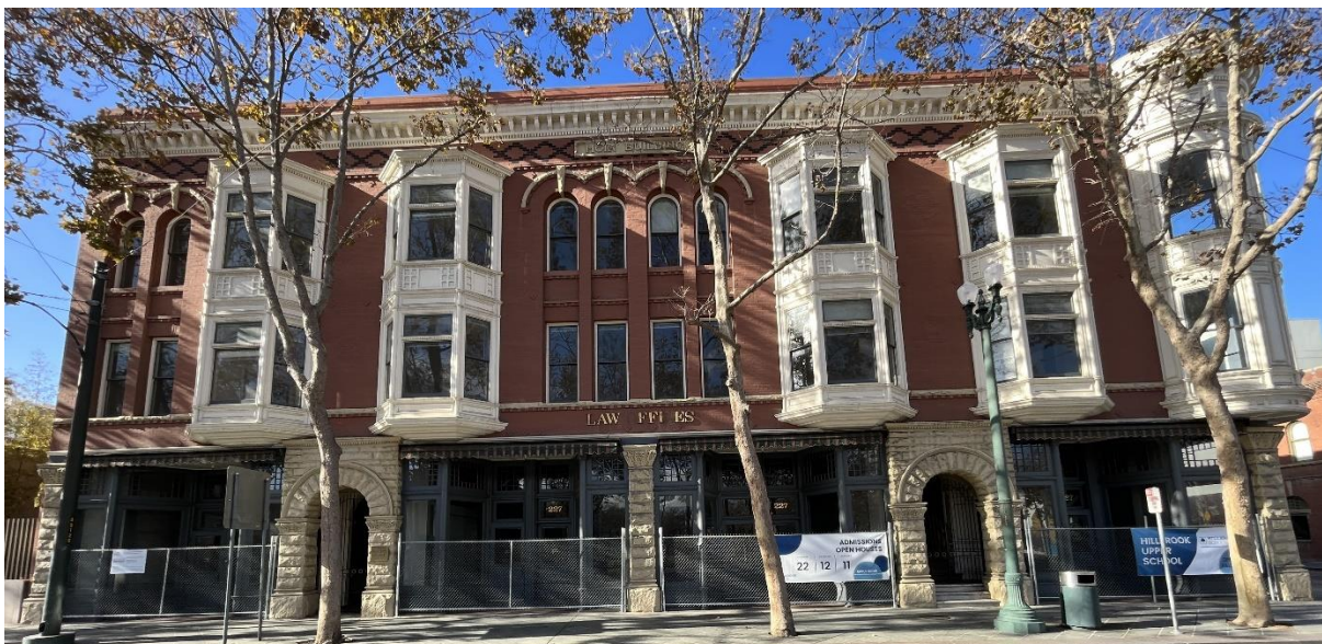
Figure 6. The east (main) façade of 227 N. First Street.
