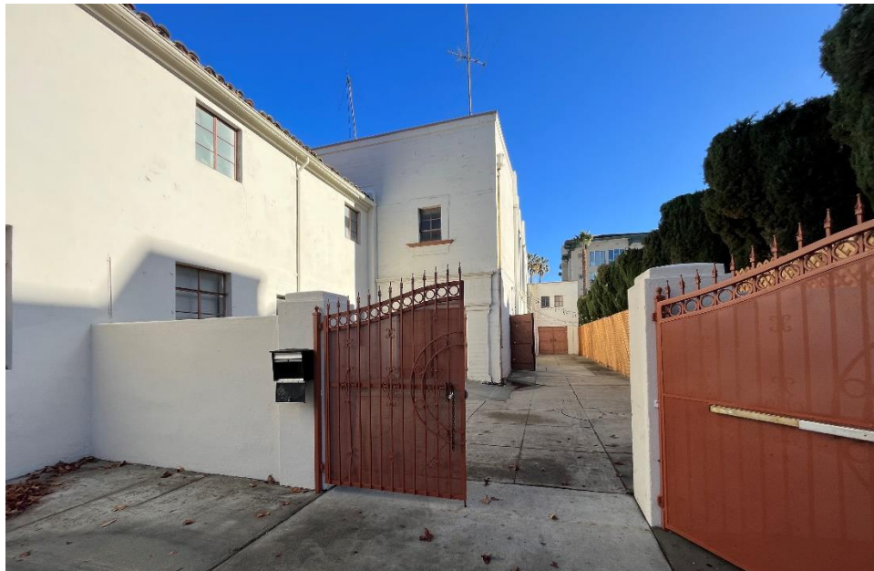
Figure 3. A partial view of the south façade of 240 N. Second Street.
