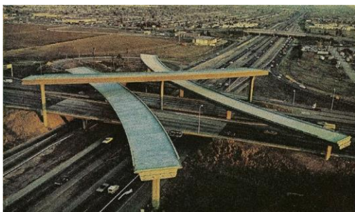
Figure 10: The 680, 280, and 101 freeway interchange, under construction in 1976
